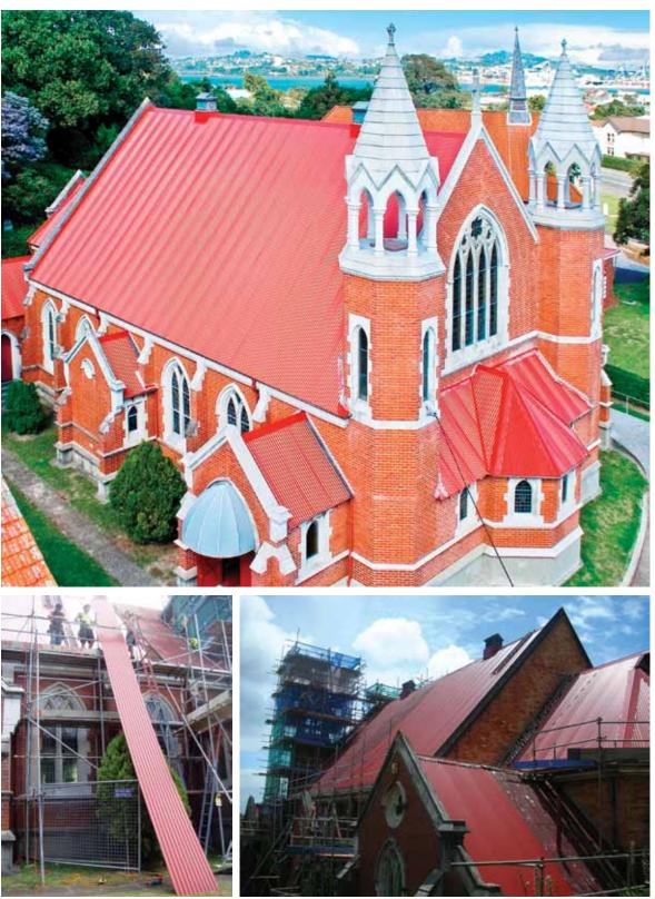
demanding physically with every single sheet having to be loaded into position by hand due because no machinery could be deployed. Metro roofers Callum Page, Ken McDonald and James Rutten, using rope harnesses, managed to install six sheets per day on the 55 degree pitch roof. EcoFleece insulation was installed where it was possible to still leave a 20mm air gap across the entire roof.
